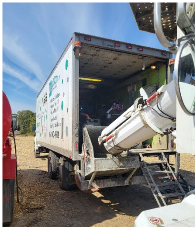
Cellular Concrete - Existing Pipe Abandonment
