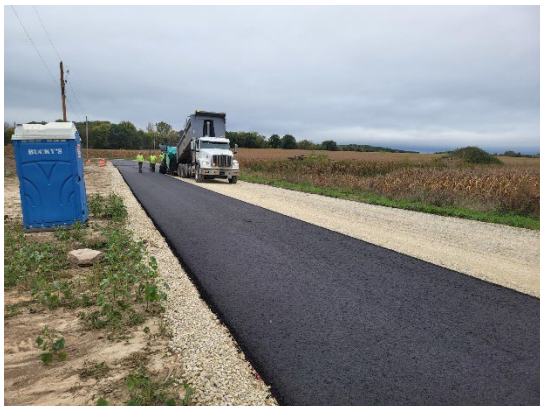
Kennedy Drive Asphalt Paving
