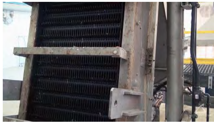
A barscreen removes large objects at the entry of Empire Wastewater Treatment Plant
