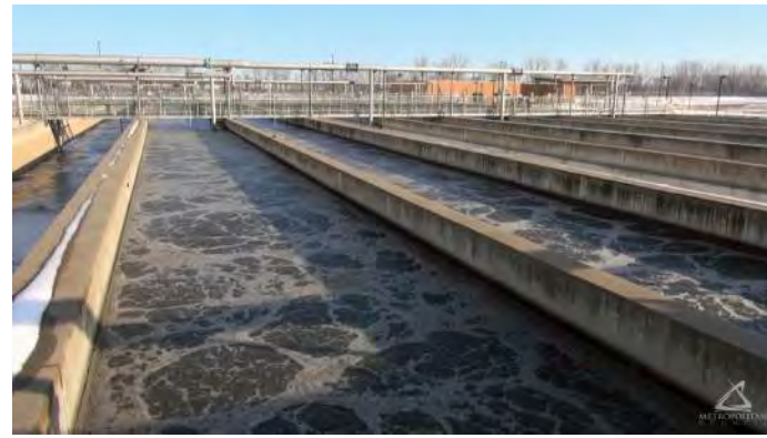
Aeration tanks at Metropolitan Council's (Minnesota) Empire Wastewater Treatment Plant create a thriving environment for bacteria to break down nutrients in the water.
