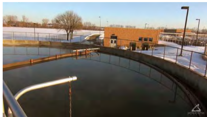
A primary clarifier allows heavy solids in the wastewater sink and fats, oils, and greases float to the top at Empire Wastewater Treatment Plant. At this plant, the biosolids are processed and applied to agricultural fields as fertilizer.
