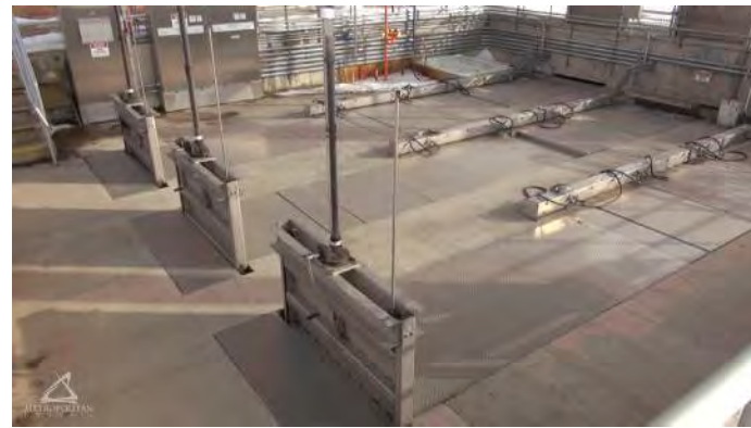
UV channels at Metropolitan Council's (Minnesota) Empire Wastewater Treatment Plant operate April through October to disinfect treated wastewater before it is returned to a local river.
