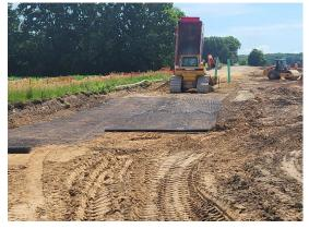
Replacing Kennedy Dr. – Placing Base Course. Geogrid placed in wet area to add stabilization.
