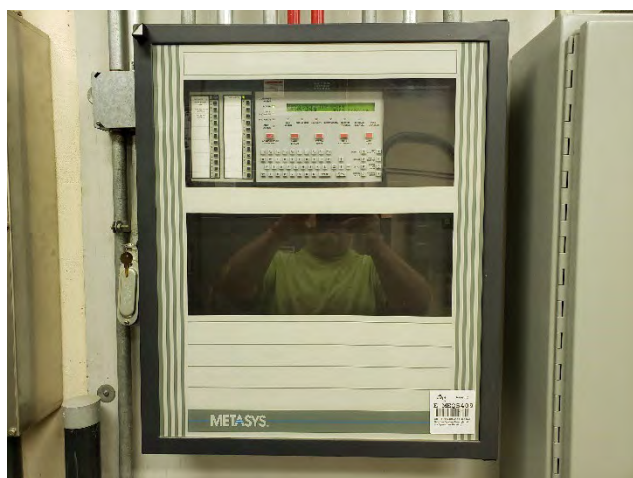
Small Johnson Controls Panel, Operator Entry
