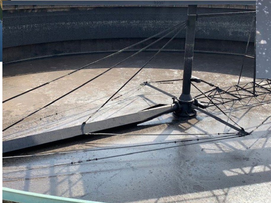
Final clarifier “TowBro” withdrawal manifold before wash-down
