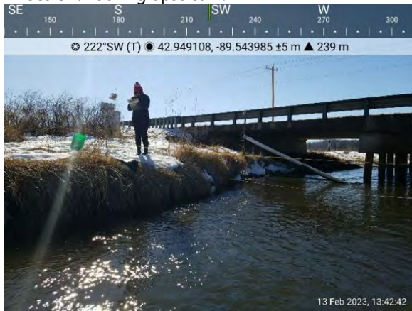
Photo 39: Looking at right stream bank.
