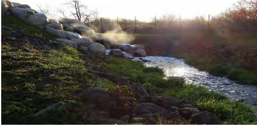
Photo 1 - Cascade Aerator at Badger Mill Creek
