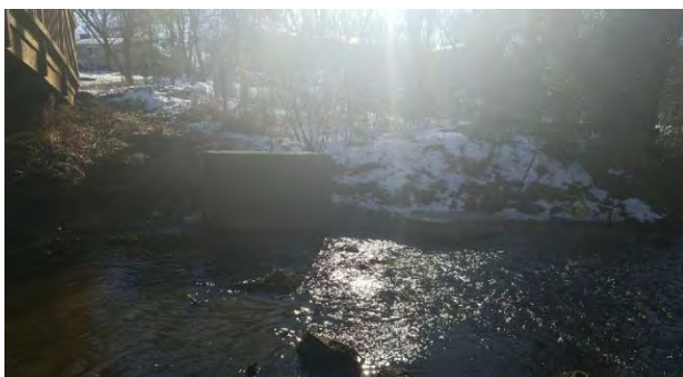
Photo 11: Looking at right stream bank.
