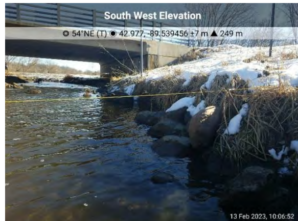
Photo 15: Looking at right stream bank.
