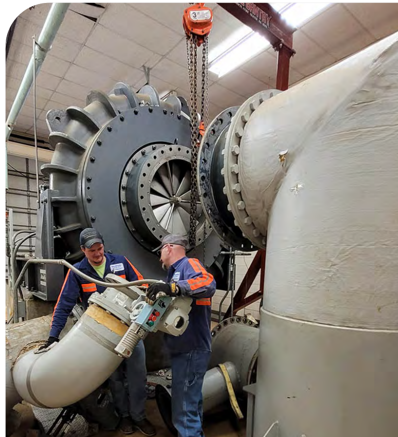
Mechanics Matt Barrett and Brian Suchomel conduct repairs on West Blower 1. Blowers pump compressed air through diffusers in the aeration tanks to ensure a continual supply of dissolved oxygen for microbes.
