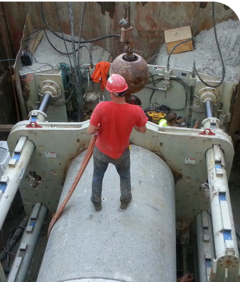
Installing replacement and relief sewer as part of the West Interceptor System project helps address additional capacity needed from recent development in Middleton and the Town of Westport.
