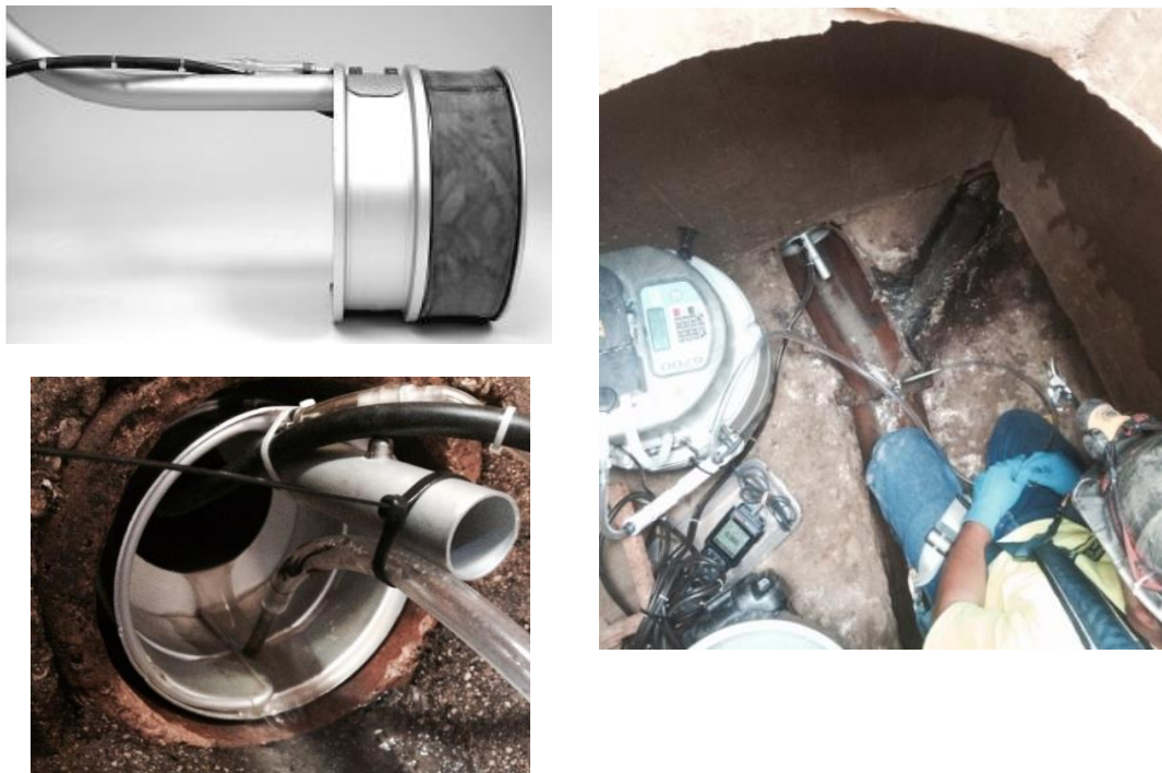
Figure 5 ISCO Flow Insert - Phase 2 Monitoring Equipment
