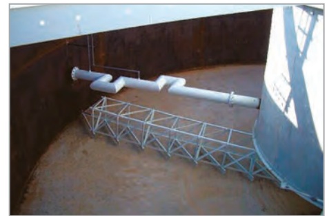
Chemical Mixing and In-line Dispersion Units
