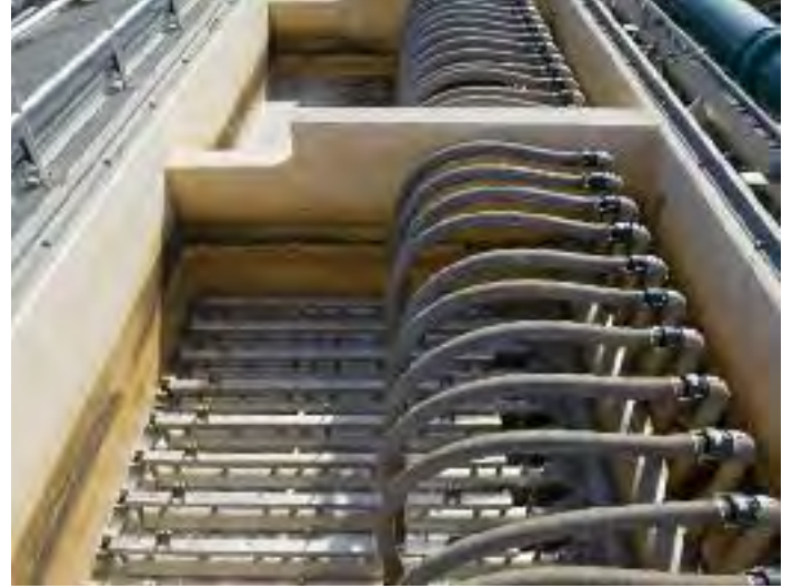
MEMCOR® Submerged membrane system
