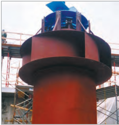
Centrifugal Impeller Pump and Draft Tube
