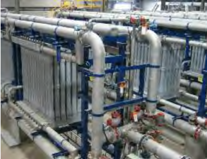
MEMCOR® Pressurized membrane system
