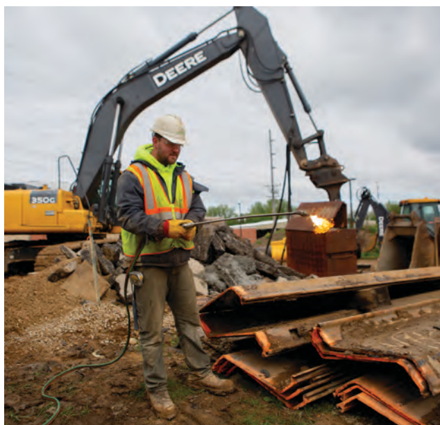
A contractor prepares to weld together components outside the Headworks Building as part of the modifications to the influent force mains to this facility.
