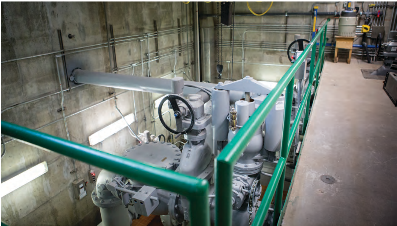
Pumping stations (also called lift stations) are used to move wastewater to higher elevations in order to allow transport by gravity flow.
