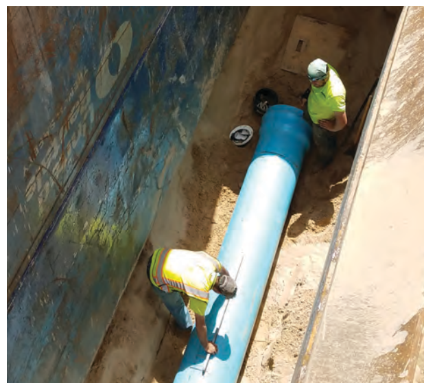
The NSVI-Morse Pond Extension consists of approximately 3,200 feet of new sanitary sewer.
