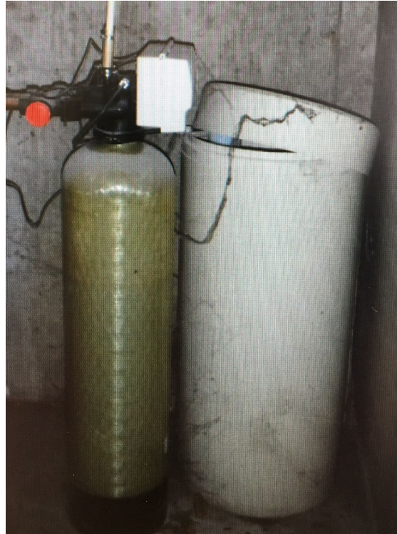
Old, deteriorated softener Efficiency: 2000 grains/pound
