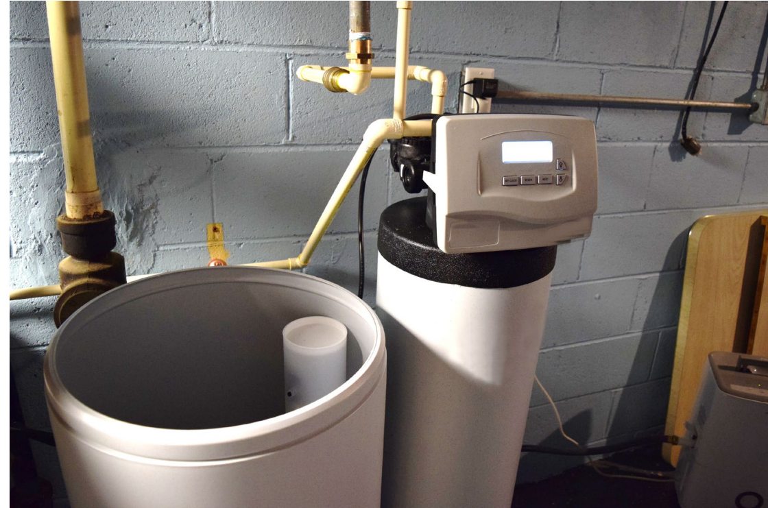
Brand new softener Efficiency: 4000 grains/pound → Can go twice as long between regenerations → Uses half as much salt
