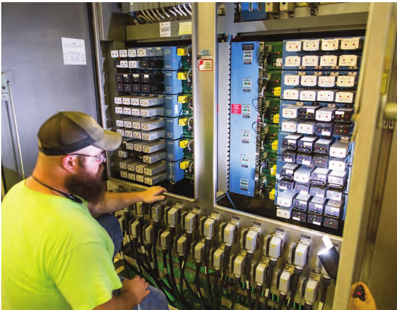
Relief Operator Cory Pieper inspects the ultraviolet power supply.
