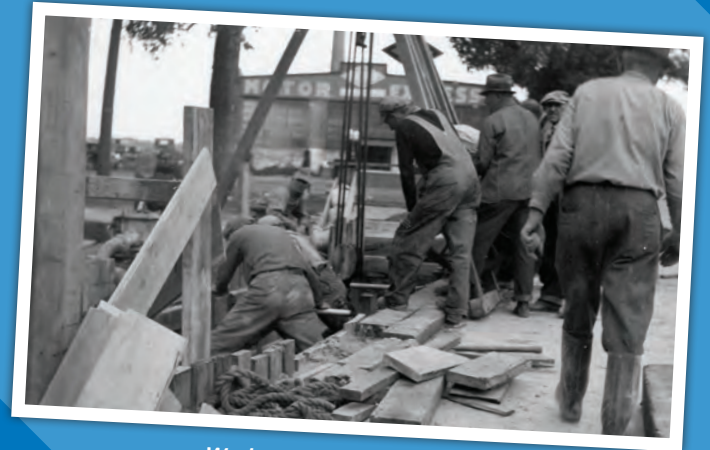
Workers lower pipe into a trench during original construction of the northeast interceptor.
