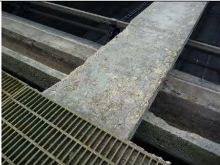
Photo 9 Primary Tank 1 top of walkway.
