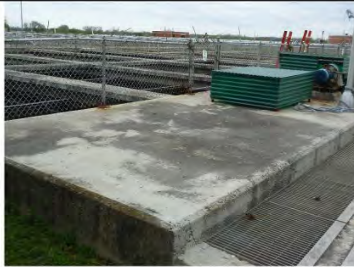
Photo 8 Primary Tank 1 top of elevated slab.
