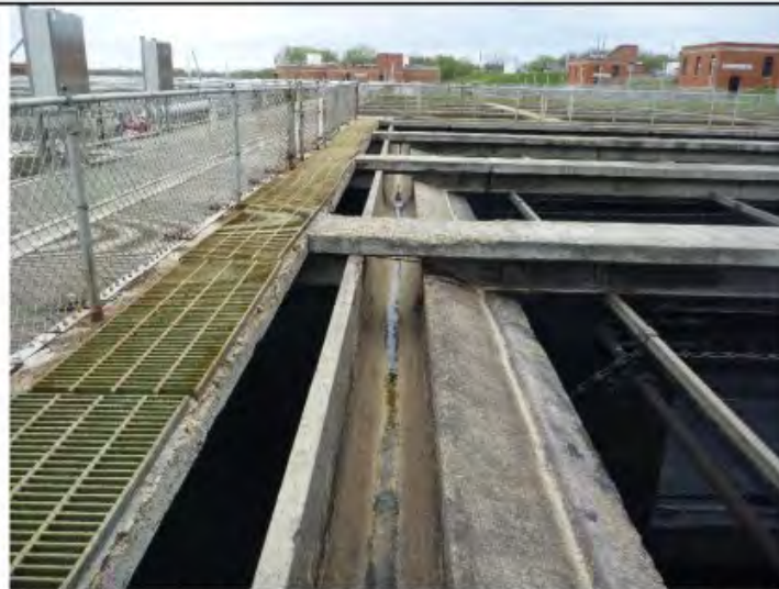
Photo 10 Primary Tank 1 edge of elevated slab.
