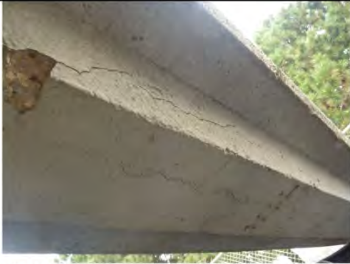
Photo 7 Primary Tank 1 bottom of walkway.
