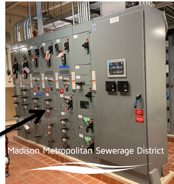
Typical new motor control center and controls
