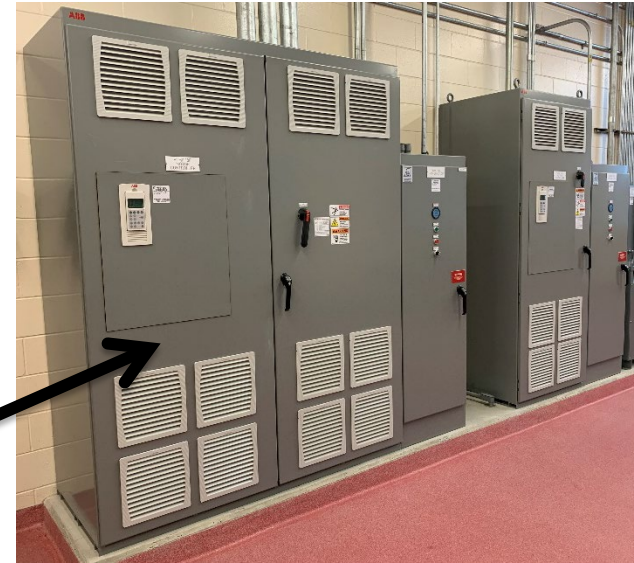
Typical new pump starters
