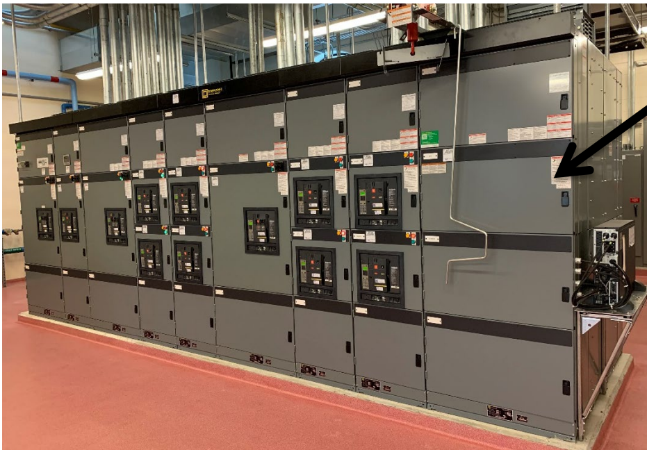
Typical new motor control center and controls
