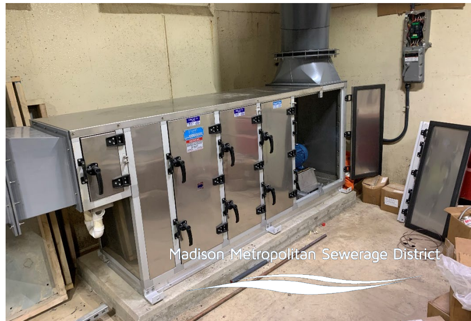
Typical new odor control unit
