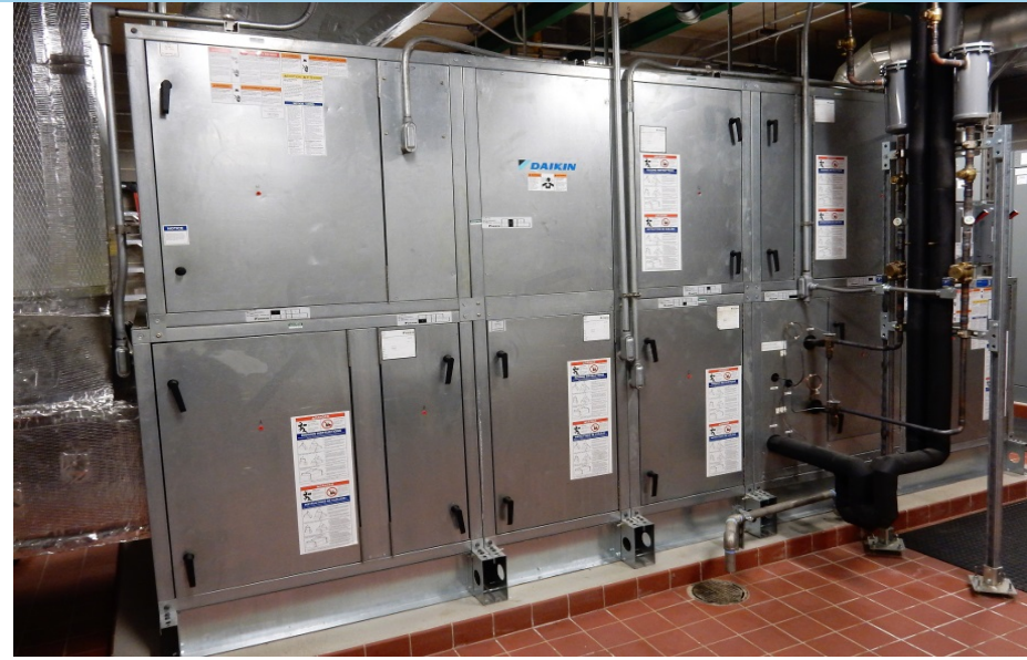
Typical new air handling unit
