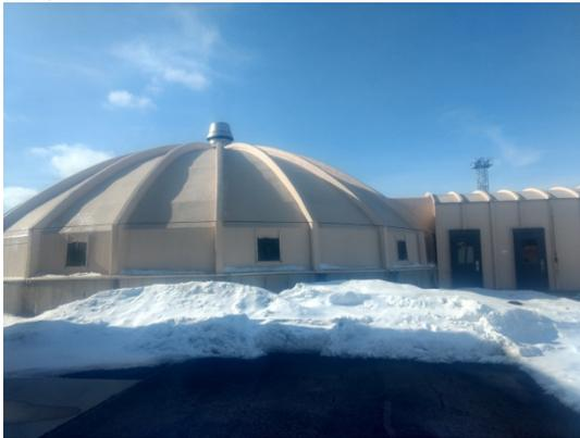
Dissolved air floatation (DAF) thickener 1 has an exhaust fan located on the peak of its fiberglass dome. This exhaust fan serves as the HVAC system for the thickener tank and provides the necessary air changes to protect equipment. Air is pulled in at the base of the dome by the fan and exhausted out of the top of the dome.
