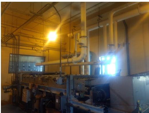
The GBT building was constructed in the late 1980's and the HVAC system remains original. Currently there are two air handling units (AHU) that serve the building; one AHU serves the polymer room and basement and the other AHU serves the belt room. There are also 4 exhaust fans that complete the HVAC system in the building. Although functional, these units are past their useful life and need replacement.
