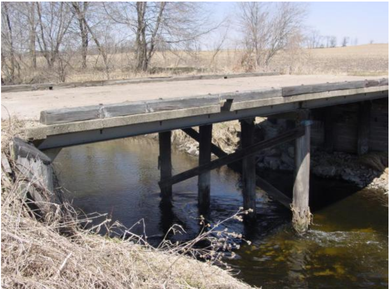
Badfish Creek Farm Bridge — The Old
